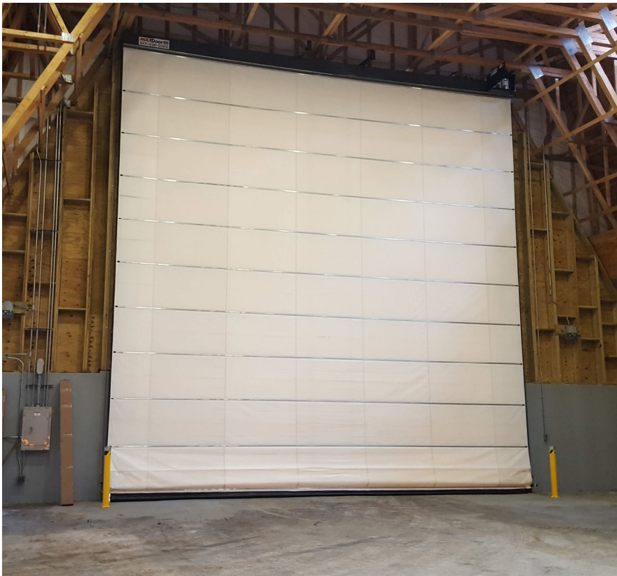
30' wide x 30' high MAXDOOR Model SD in Timber Construction Building
